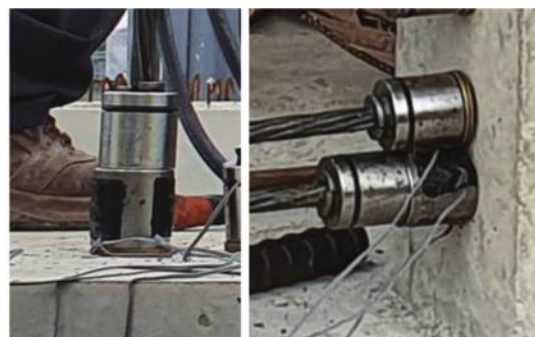
(a) Anchorage of vertical and horizontal tendons
