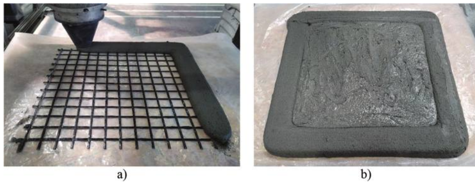
Fig. 5—Demonstration of process of creating a slab: (a) 3-D printing of slab contour; and (b) contour filled with concrete.
