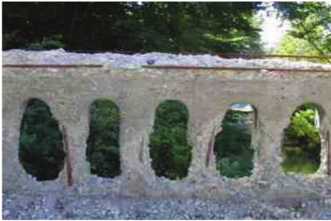
Fig. 2—Buildings damaged due to F&T effect (Paul 2014).
