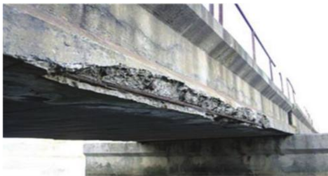
Fig. 5—Corrosion-induced damage on Cape Town concrete bridge exposed to airborne chlorides (Alexander and Beushausen 2019).
