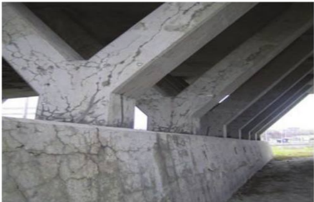
Fig. 4—Du Vallon-Charest highway interchange viaduct, Québec, QC, Canada, was recently demolished because of alkali-silica reaction (Fernandes and Broekmans 2013).
