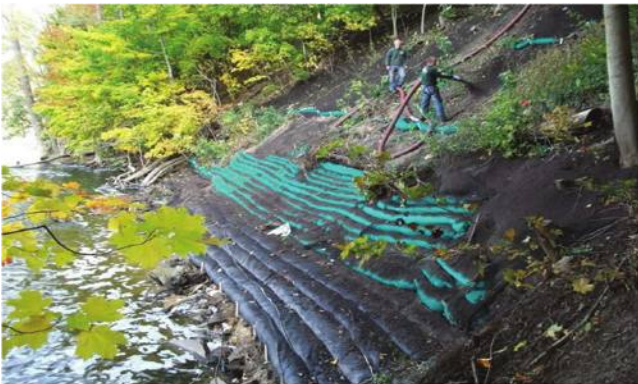
Fig. 4—Beach erosion control by using erosion control blankets.
