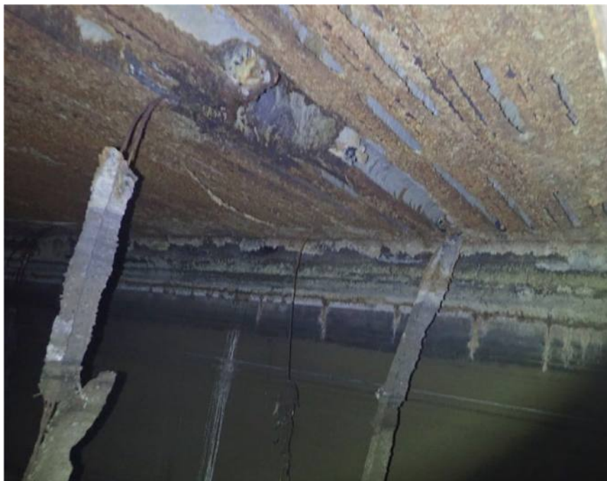
Fig. 3—Soffit of precast roof panels with hollow cores exposed due to BSA activity.
