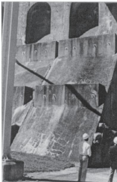
**Figure 6.3** Cracking caused by alkali–silica reaction.
