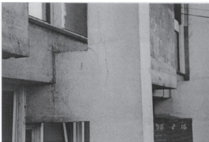
**Figure 6.1** Structural cracks at a column beam connection.
