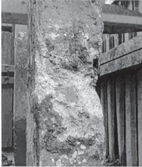
**Figure 6.5** Foundation damaged by thaumasite attack.
