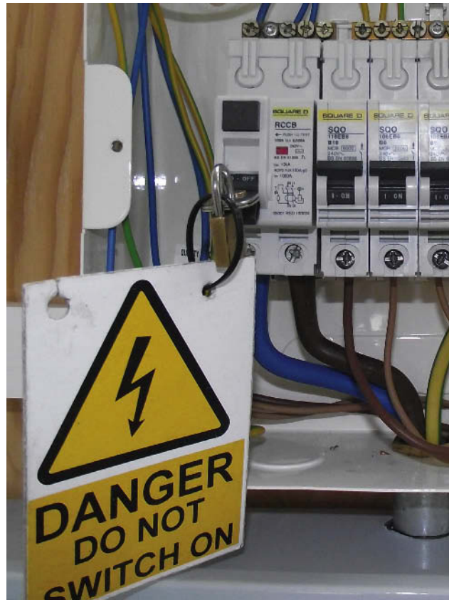
Figure 4.25 Always ensure that circuits are 'locked off' before working on them.
