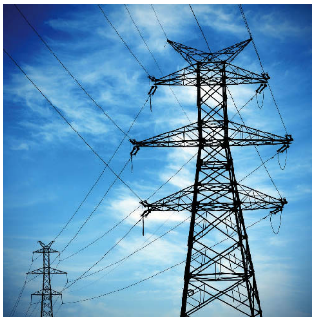
Figure 3.10 Transmission line steel pylon.
