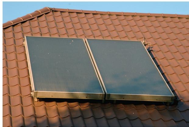
Figure 11.10 Flat plate solar thermal panels.
