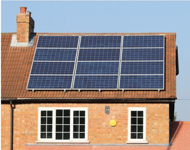
Figure 11.14 Monocrystalline PV array.
