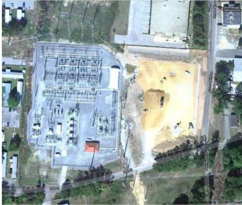
Photograph 1 Aerial View of Existing Substation and Expansion Area (Google Maps 2012)
