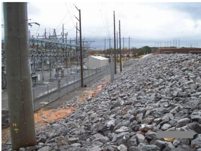
Photograph 5 Slope Between Existing Substation and Expansion Area
