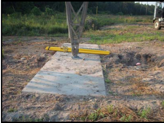
Photographs 21 and 22 – Completed Micropile Mat Foundations with Temporary Supports Removed
