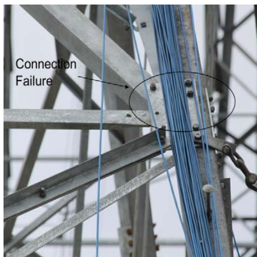
Figure 15 - Failed connection
