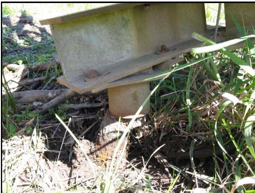
Photograph 5 – Middle Phase Tower Foundation
