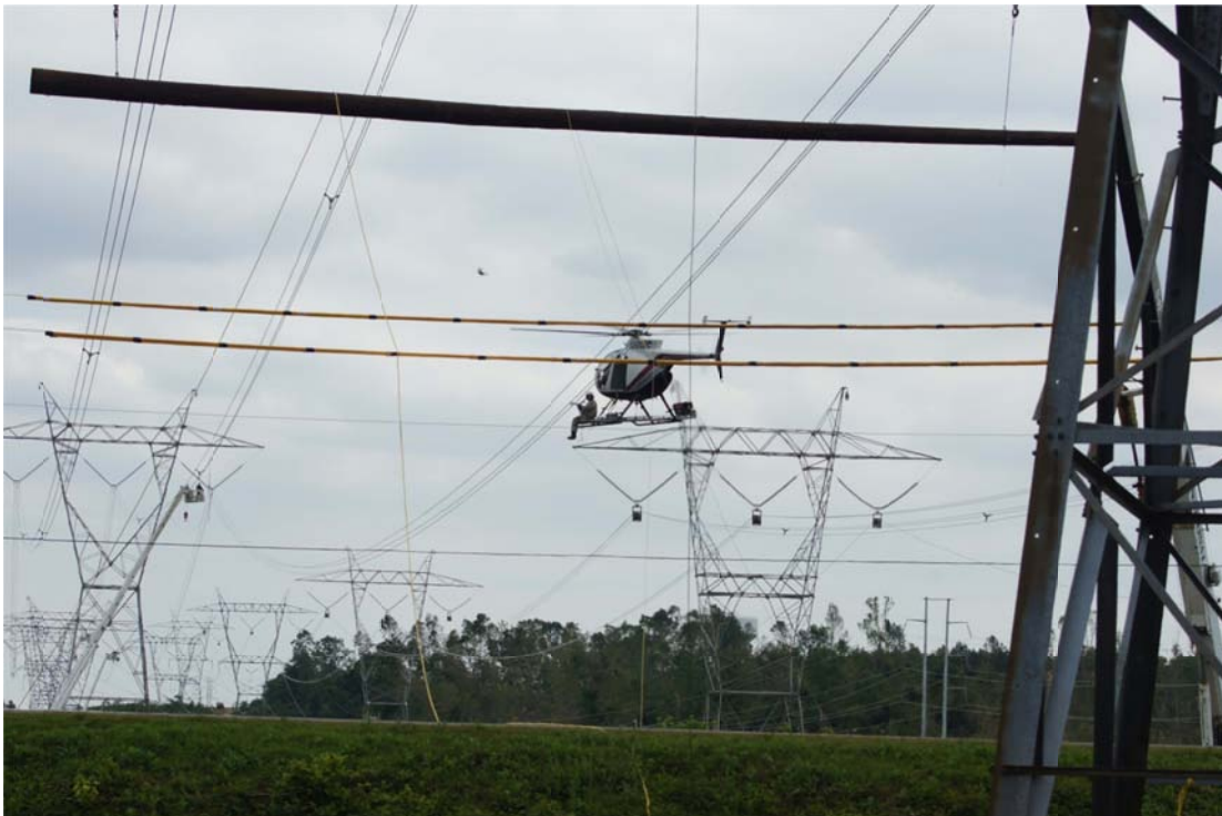
Figure 6. 500-kV restoration utilizing helicopter support (courtesy of TVA)
