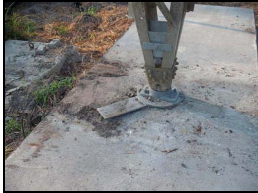
Photographs 21 and 22 – Completed Micropile Mat Foundations with Temporary Supports Removed
