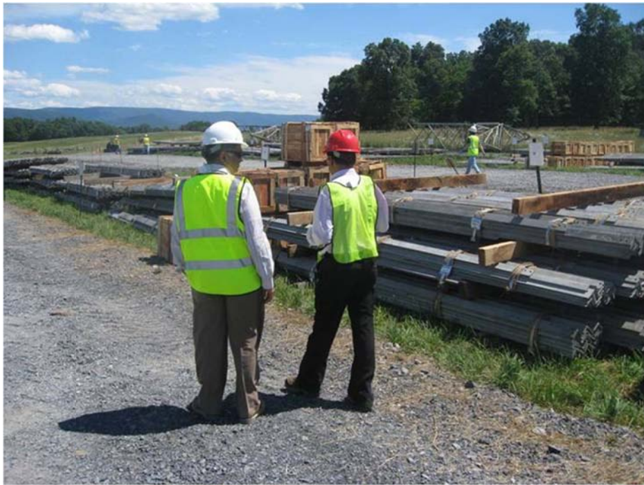
Photo 1. Old Fields Material Yard
