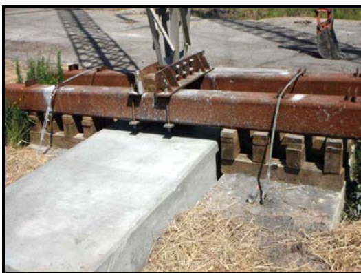
Photographs 19 and 20 – Concrete Mat Construction Complete with Temporary Supports Still in Place
