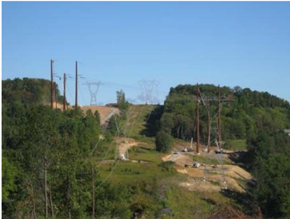
Photo 4. Tubular Steel used for 500kV crossing
