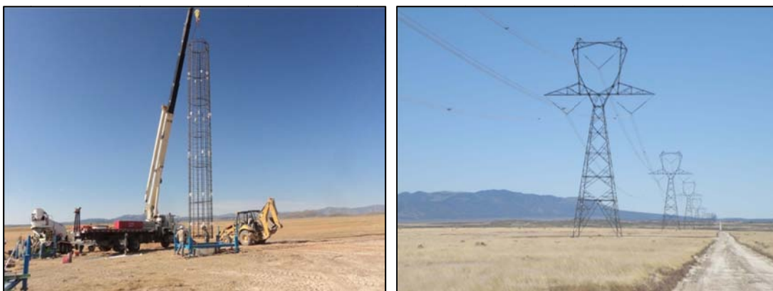
Figure 8. Foundation installation and completed towers in Tooele County, Utah.
