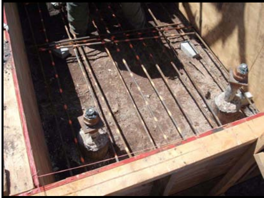
Photographs 15 and 16 – Concrete Mat Foundation Micropiles and Reinforcing
