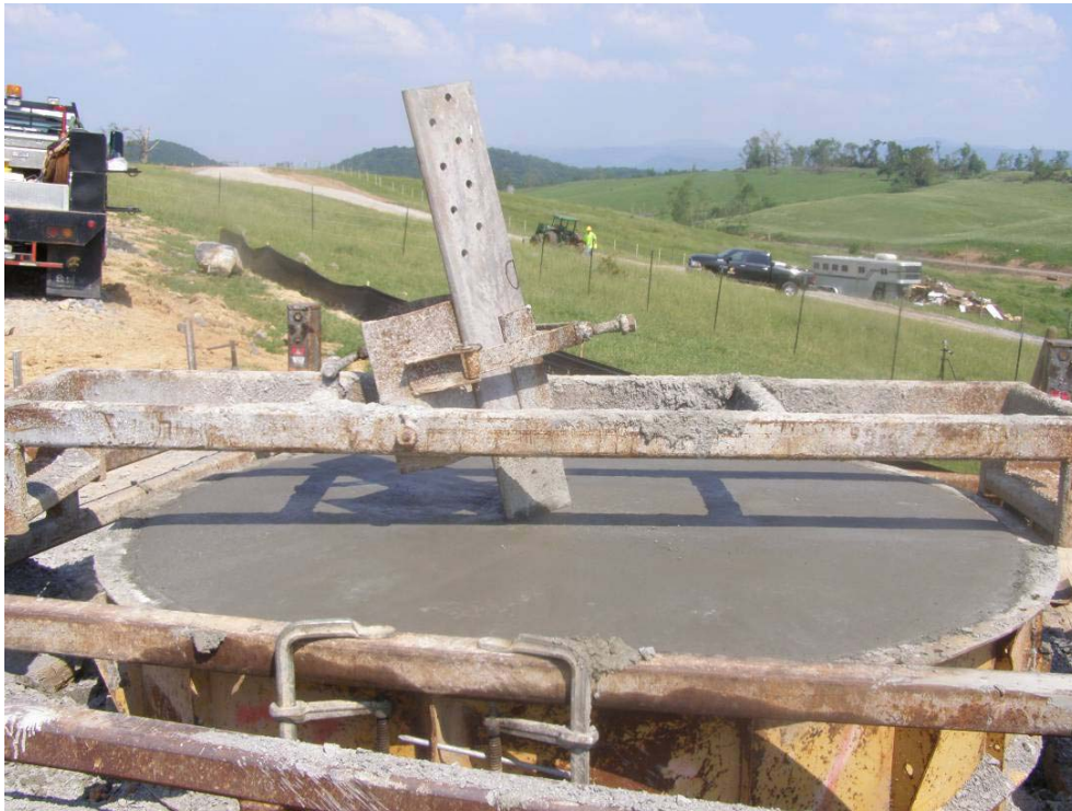
Figure 6 – Concrete Form with Stub Jack and Positioner
