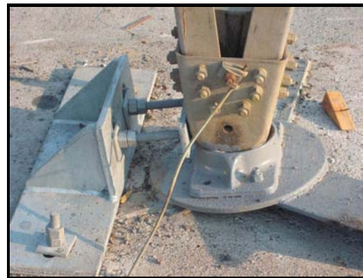
Photographs 23 and 24 – Middle Tower Completed Foundations with Cup Retainer Bracket
