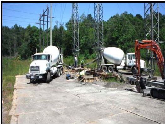
Photographs 17 and 18 – Concrete Mat Construction
