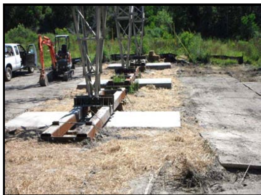
Photographs 19 and 20 – Concrete Mat Construction Complete with Temporary Supports Still in Place
