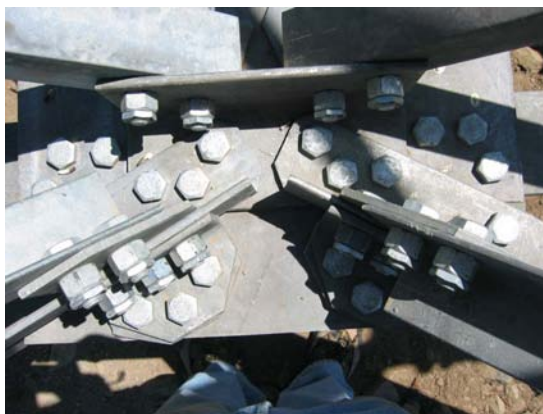
Figure 2. Complex Member Connection Detail (Courtesy of BPA)
