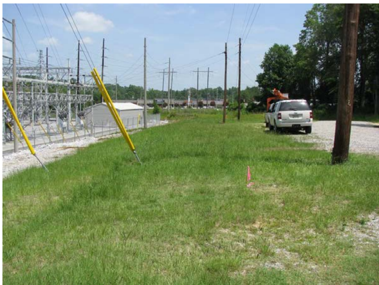
Photograph 2 Expansion Area Prior to Construction
