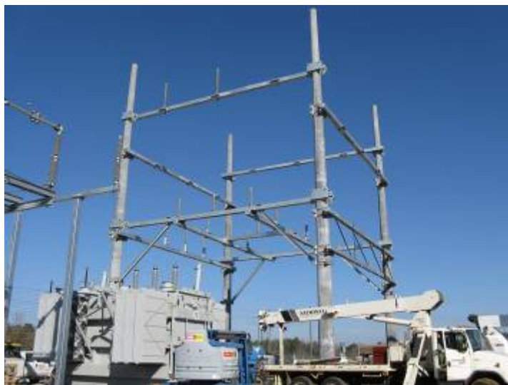
Photograph 6 Construction of Concrete Pole Structure
