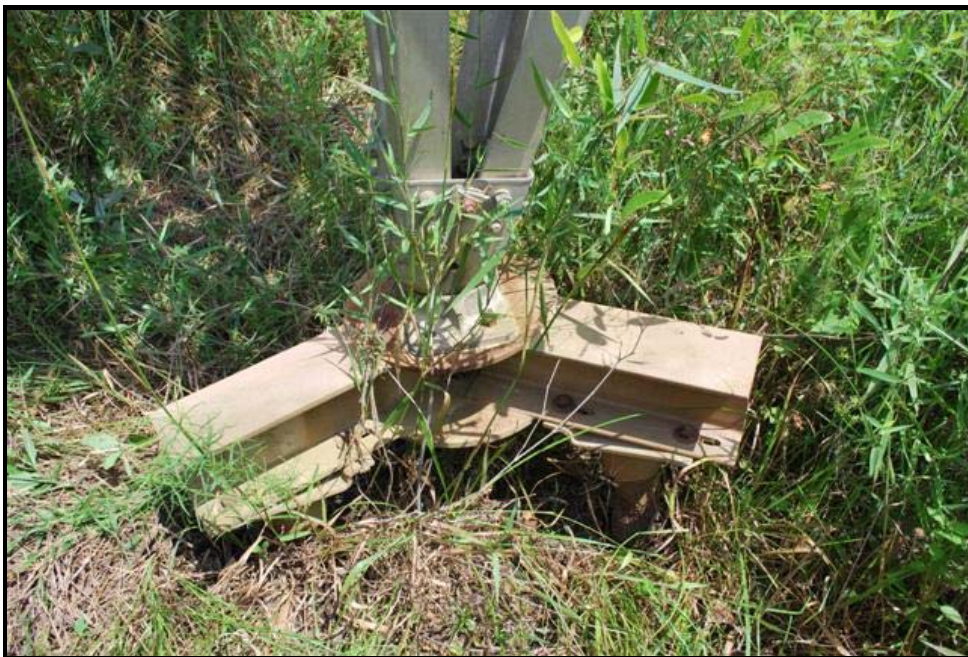
Photograph 2 – Helical Anchor Grillage Foundations
