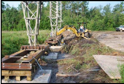
Photographs 6 and 7 – Temporary Steel Framing and Foundations
