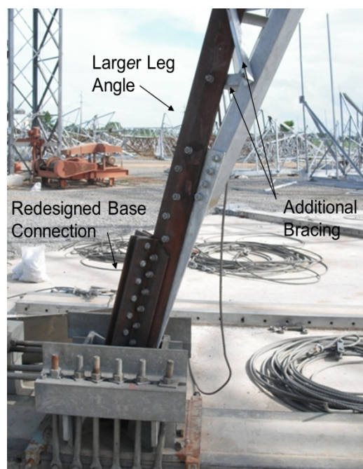
Figure 10 - Base connection revised
