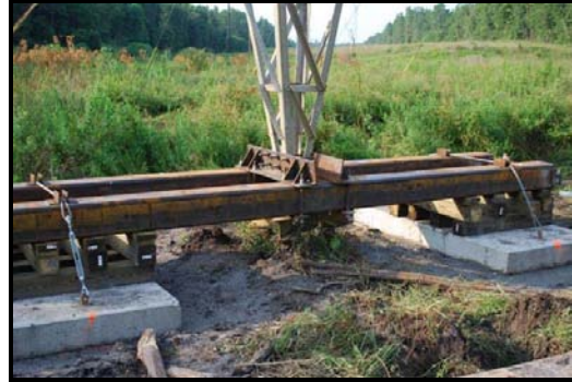
Photographs 6 and 7 – Temporary Steel Framing and Foundations
