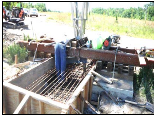
Photographs 15 and 16 – Concrete Mat Foundation Micropiles and Reinforcing
