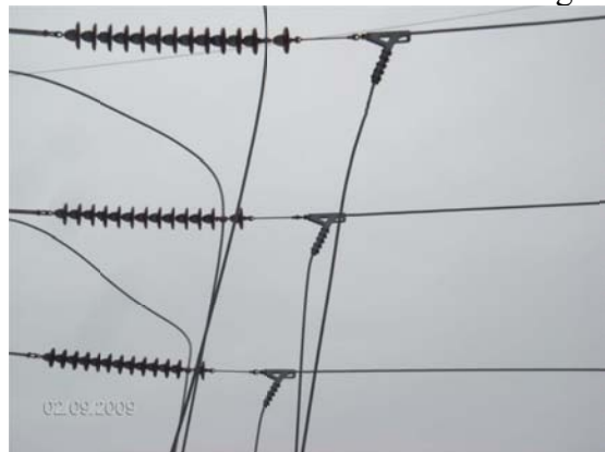
Photograph 4 – Addition of Extensions at Terminal Structure to Provide Extra Sag
