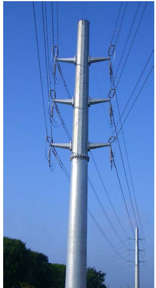
Photo 4 – Multisided top and roll formed bottom Photo Courtesy Valmont Newmark
