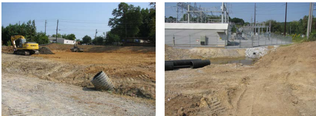
Photograph 3 and 4 Expansion Area During Construction
