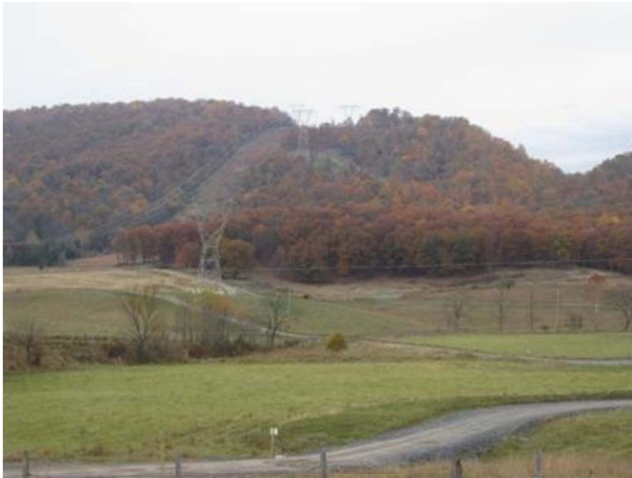
Photo 2. Example of Selective ROW Clearing
