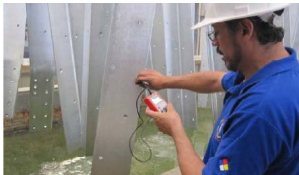
Figure 4 - Measuring the thickness of galvanizing (Photo courtesy Southern California Edison)
