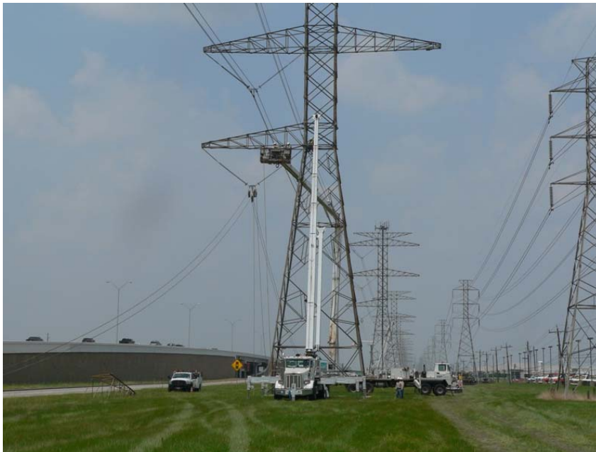
Figure 2. Restoration Using Empty Circuit Arms
