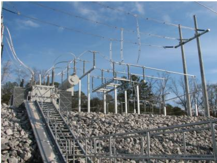
Photograph 11 Expansion Area after Construction
