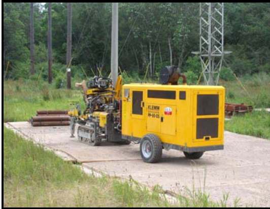
Photographs 10 and 11 – Micropile Installation
