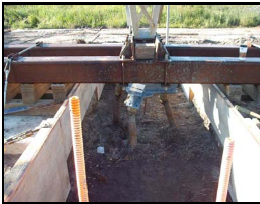
Photographs 12 and 13 – Concrete Mat Foundation Forming
