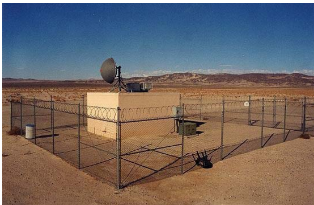
Figure 5: Control Building located at a Ground Electrode Facility (courtesy of The Center for Land Use Interpretation)
