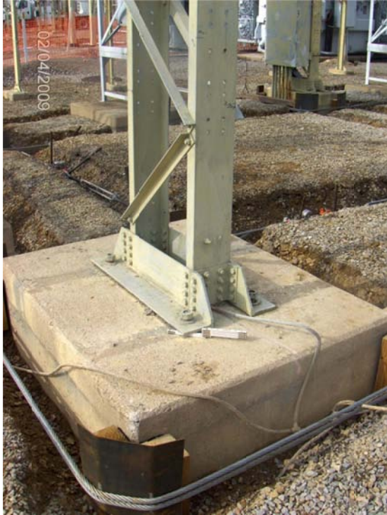
Photograph 1 – Mitigation Measures, Cable Wrapping & Monitoring
