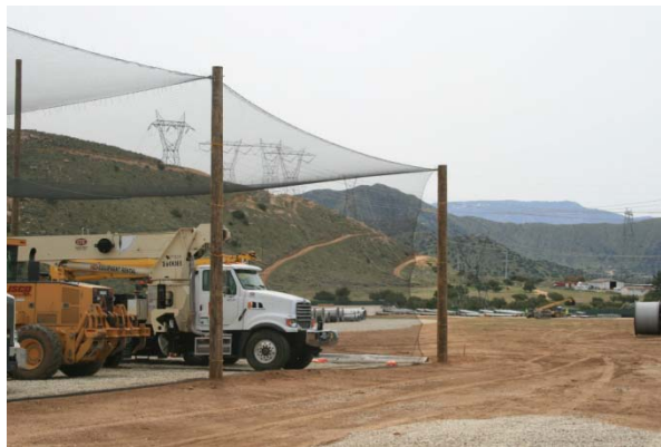
Figure 5. Netting used to prevent nesting on construction equipment (with permission from PAR Construction).
