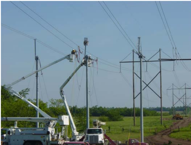
Figure 2, 345 kV Energized Reconductoring
