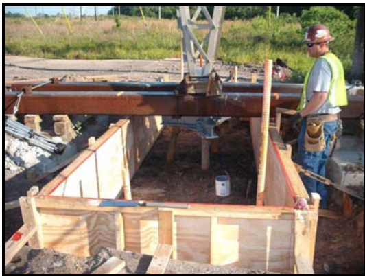
Photographs 12 and 13 – Concrete Mat Foundation Forming
