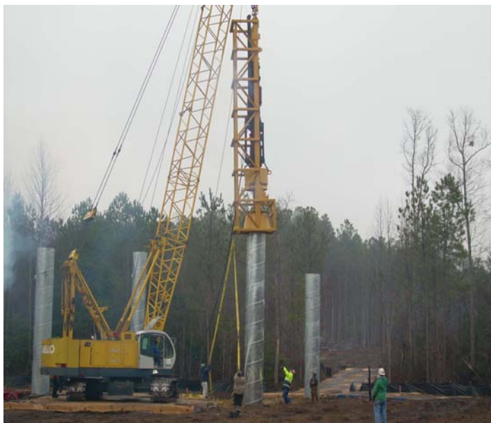
Figure 9. Photograph of Outer Pipe Pile Installation
