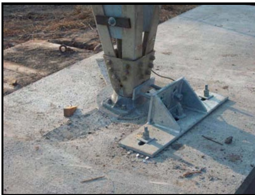
Photographs 23 and 24 – Middle Tower Completed Foundations with Cup Retainer Bracket
