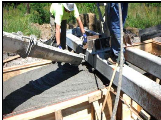
Photographs 17 and 18 – Concrete Mat Construction
