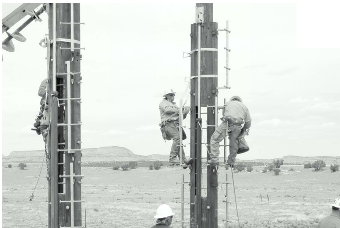
Figure 3: Installation of Phase Raiser ® Assembly is shown on a 115kV H-frame Structure. Assembly shown lifts structure six (6) feet. (Photo courtesy of PNM.)
