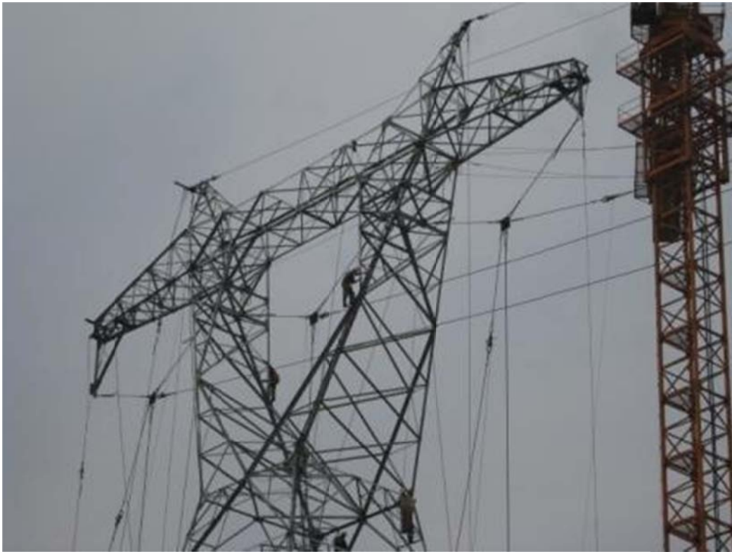
Photo3. Lattice Steel Ready for Testing
