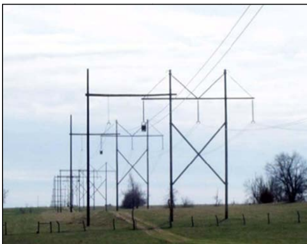
Figure 1, 345 kV Live Reconductoring
