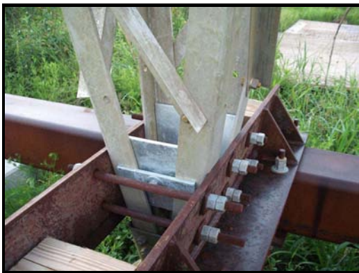
Photographs 8 and 9 – Temporary Steel Framing and Foundations
