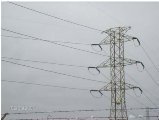
Photograph 3 – Taut Conductor to Tower 36
