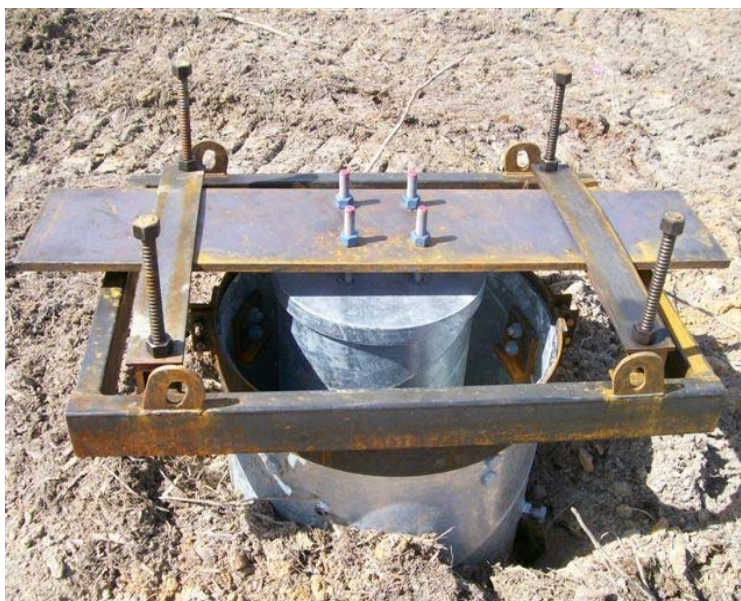
Figure 10. Completed Foundation Prior to Concrete Pour
