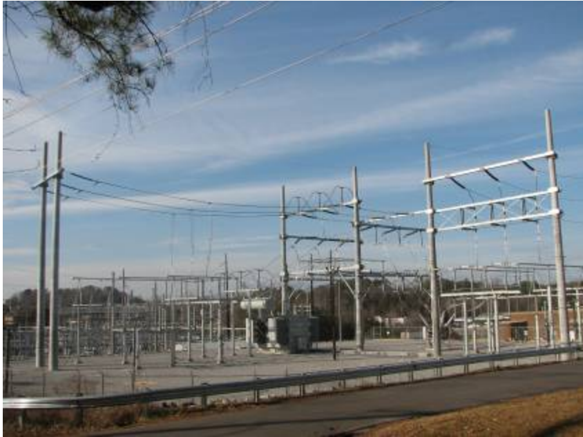
Photograph 10 Expansion Area after Construction
