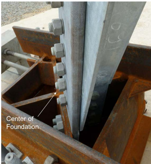
Figure 17 - Eccentricity at base
