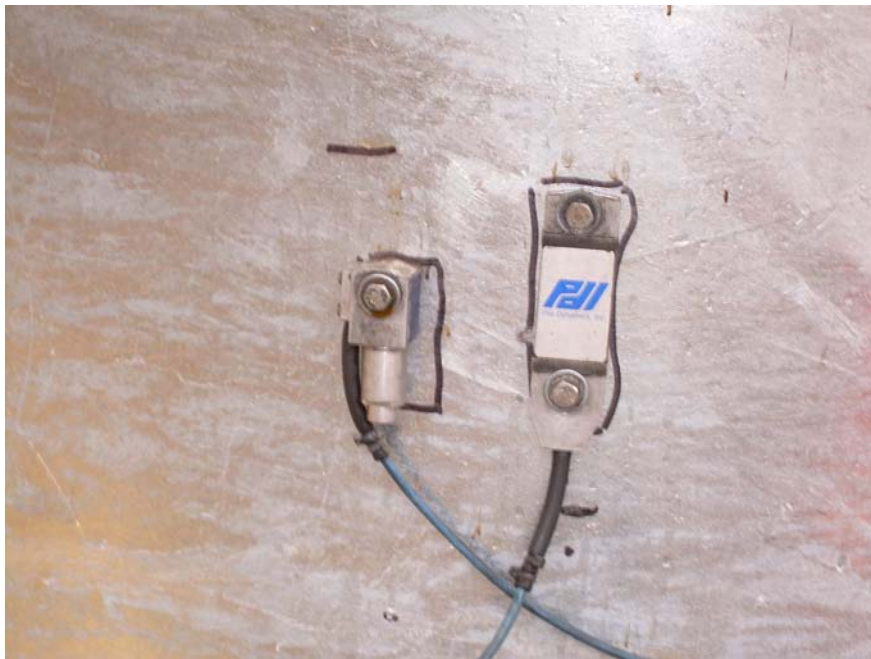
Figure 11. Accelerometer and Transducer Bolted to Pipe Pile for Dynamic Pile Testing
