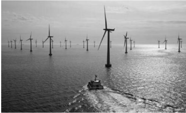
FIGURE 3.1 Wind Lillgrund offshore farm between Malmö and Copenhagen, the Netherlands. (Copyright Siemens Presspicture. With permission.)
