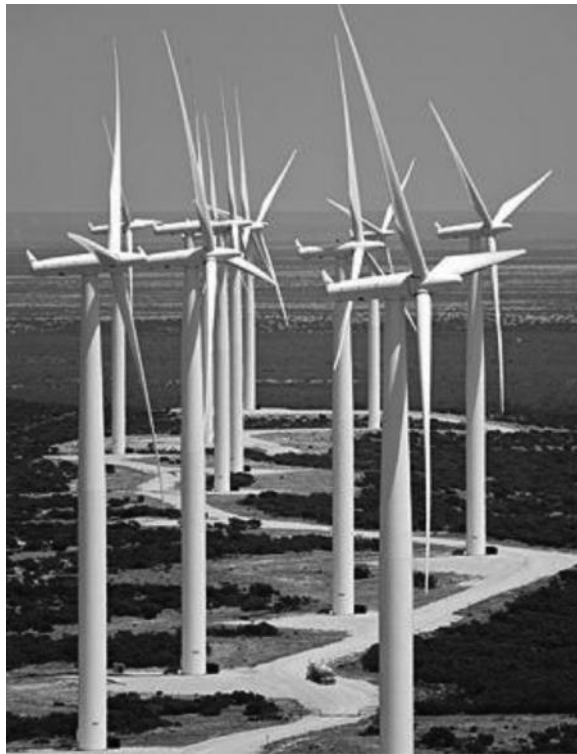
FIGURE 3.2 The elbow creek wind project near Big Spring, Texas. (Copyright Siemens Presspicture. With permission.)
