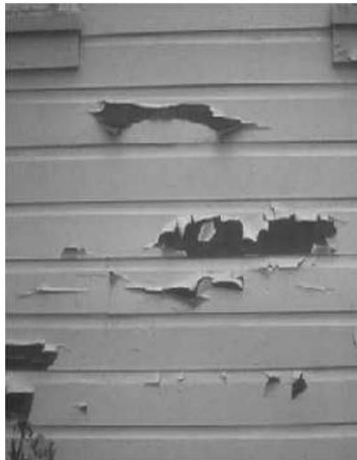
Figure 7.18 Flaking (Courtesy: Sigma Coatings)
