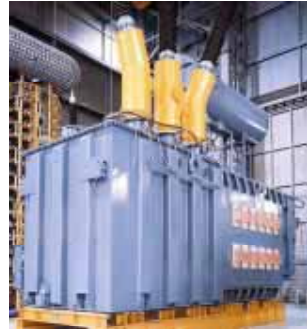
79 MVA Rectifier Transformer. Common tank.
